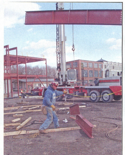
An ironworker hooks up a string of beams for the Link-Belt crane operator.
