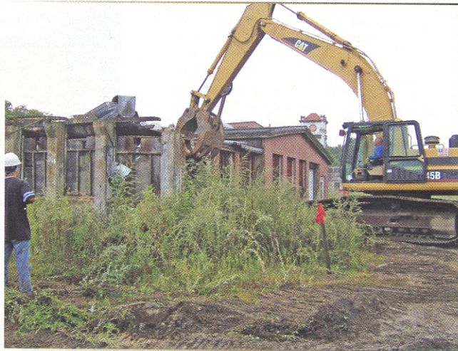
AA Wrecking Co. uses a Cat excavator equipped with a grapple to tear down old mill buildings. (D. Joubert photo)
