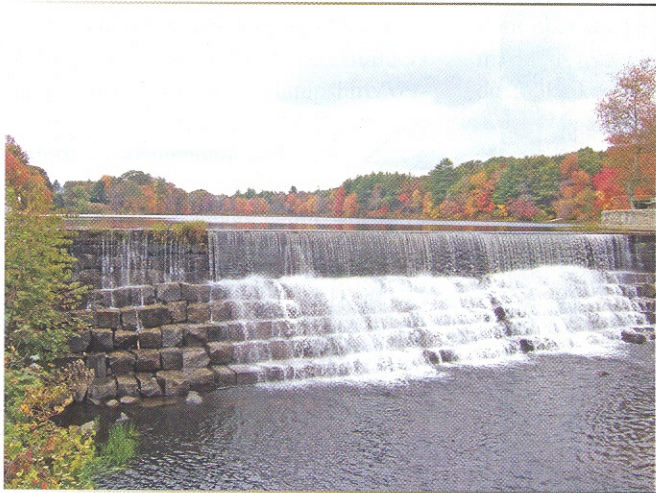
Dam built in 1850s created a pond on the Clear River to provide dependable water supply for mills. (D. Joubert photo)
