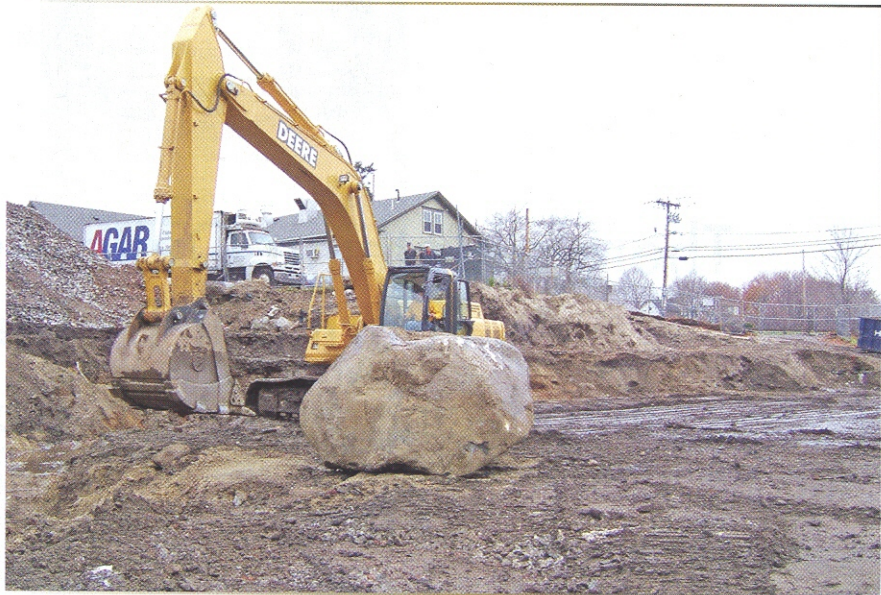
Hundreds of glacial boulders, some as big as five cubic yards, were unearthed on the site. (D. Joubert photo)
